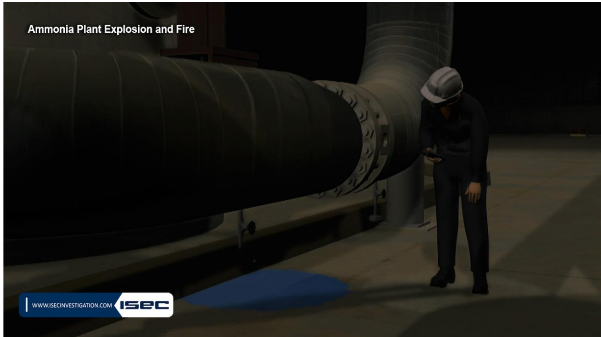
Figure 1. Leakage in 32-inch semi-lean amine pipeline
